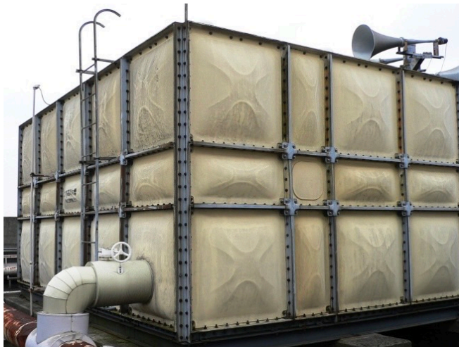
Before coating application ( FRP elevated water tank)
